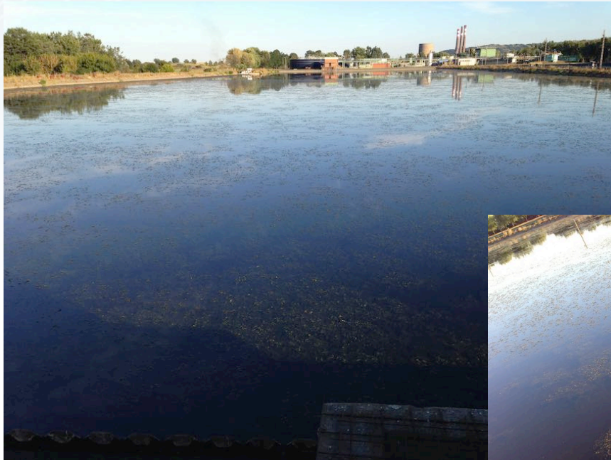
Tertiary treatment pond aquatic weed blooming before Pond Pure bioaugmentation
